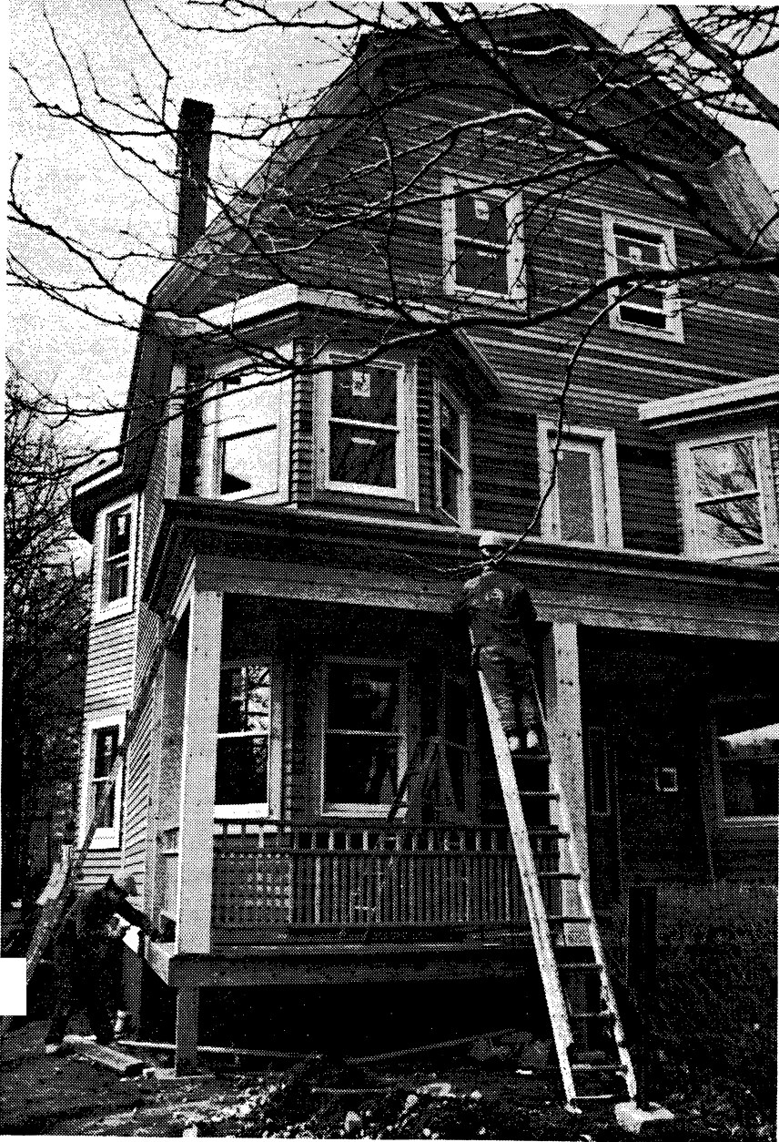
The Affordable Housing Trust provided funds to help create a group home for ten low and moderate income mentally ill adults. This architecturally attractive project builds bridges between neighbors and differently abled persons.
