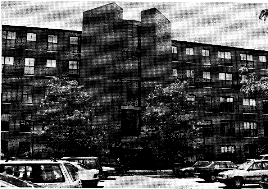
The former Henderson Carriage Factory was rehabilitated for use by a variety of occupants, including a restaurant, a bank, and several small firms.
