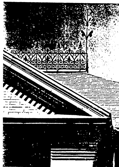
56. Clerk of Courts Addition. Exterior detail.
