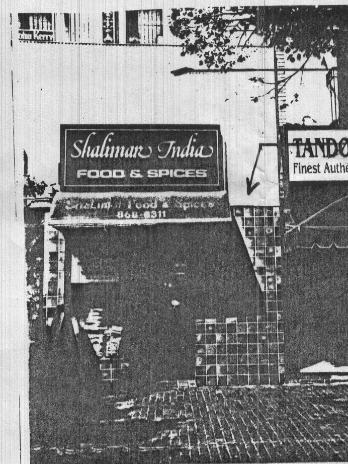
EXIST. PHOTO OF TILE PILASTER
