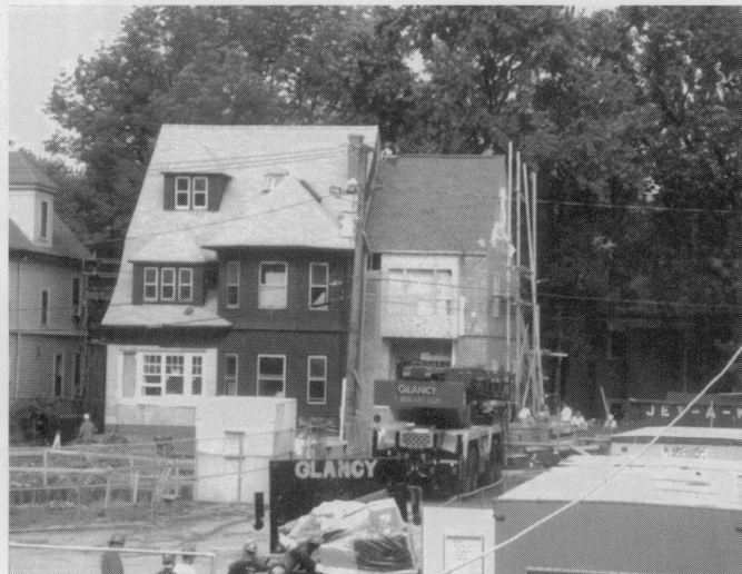
Above: Construction on the new Birth Center has been moving right along throughout the summer, and is expected to be completed before the new year.
