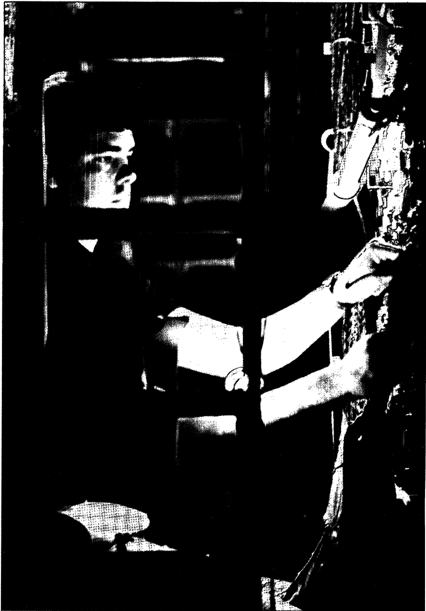
THE NETWORK GROWS: The installation of new equipment calls for special care. Each addition must be compatible with all equipment in other cities and towns so that customers can call here, there, and everywhere. David Tabb is wiring new switches to add another area to the Direct Distance Dialing network. Some 97 per cent of New England Telephone customers can dial their own long distance calls.
