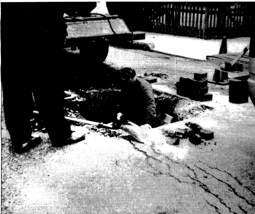
DPW Workers repair utility cover at South Normandy Avenue.
