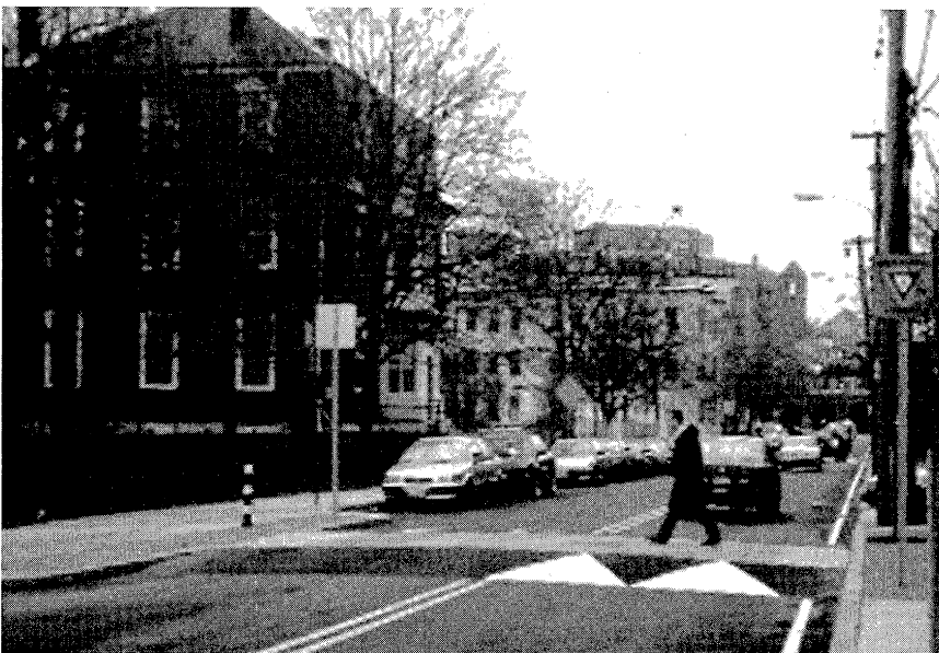
This raised crosswalk at the entrance to Columbia Street Park is one of the features of the Columbia Street Traffic Calming project completed this year.
