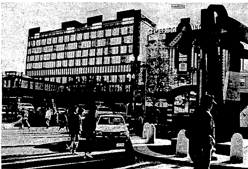
Holyoke Center, with its ground floor retail and university administrative offices above, combines business and institutional uses in one complex.
