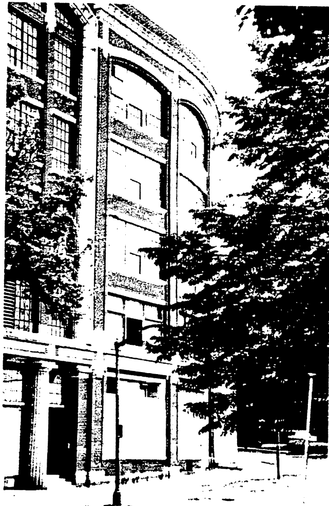
The former Ford Assembly Plant is being renovated for occupancy by a firm that specializes in personal emergency response systems.
