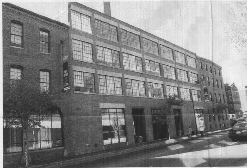
6 EXISTING CONDITIONS SCALE: N/A
