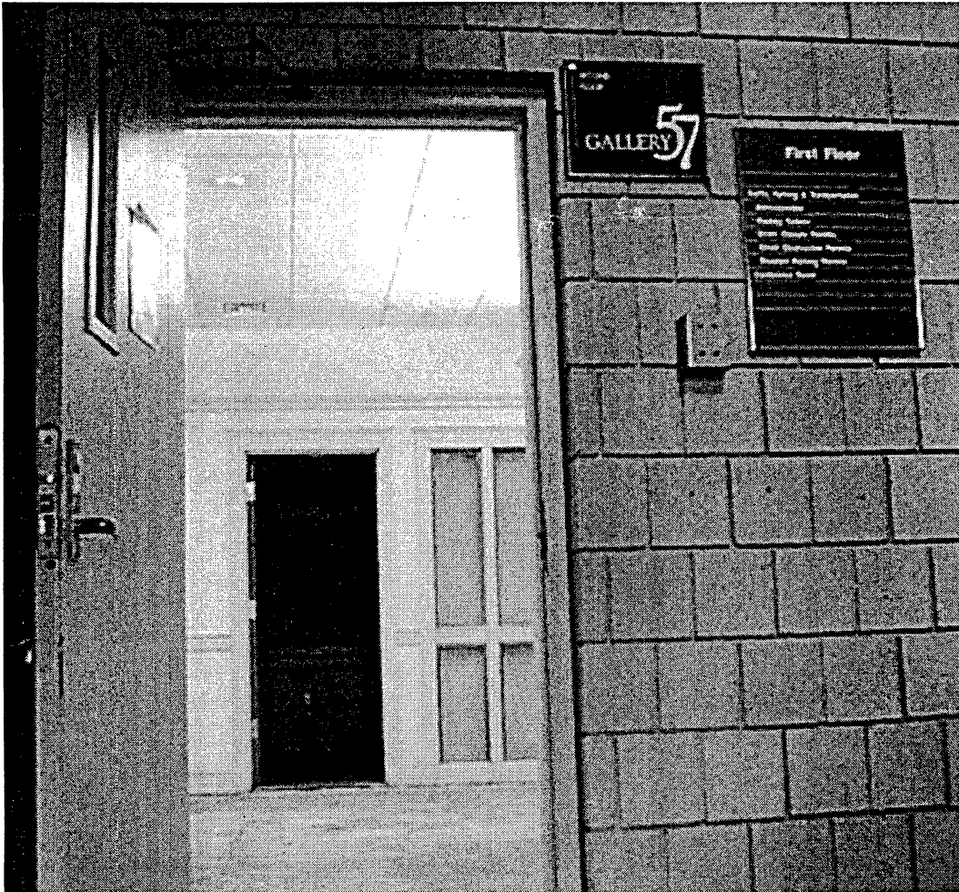
Existing Conditions: Visitors to the building enter into a stairway
