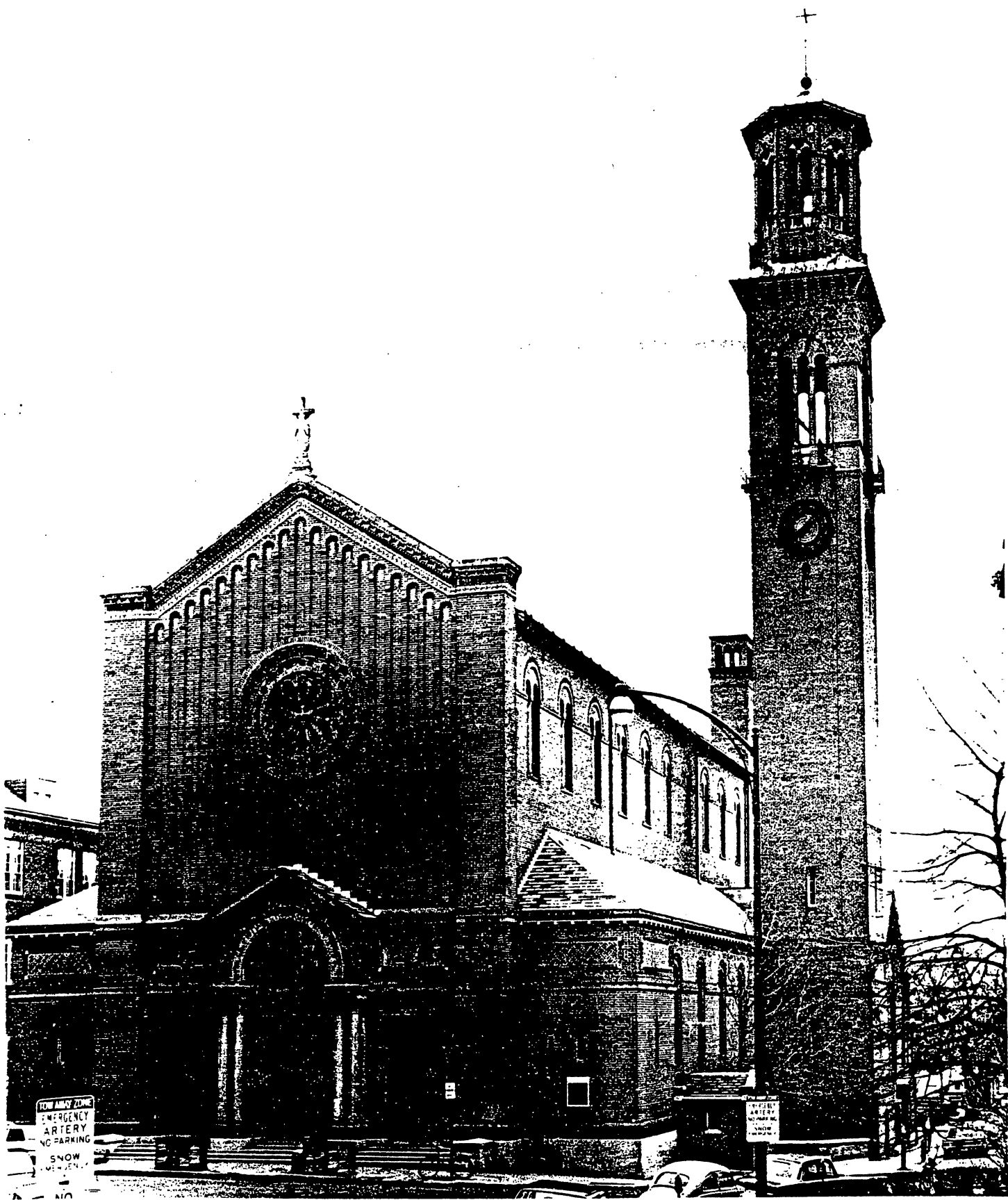
St. Paul's Roman Catholic Church, 24 Mount Auburn Street
