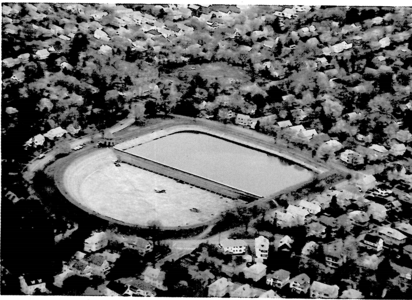
November, 1989 — The Payson Park Reservoir providing uncovered treated water to the city before construction began in the North Basin.
