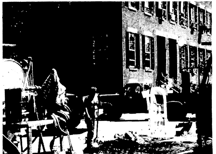
Sewer replacement — Essex Street and Bishop Allen Drive.
