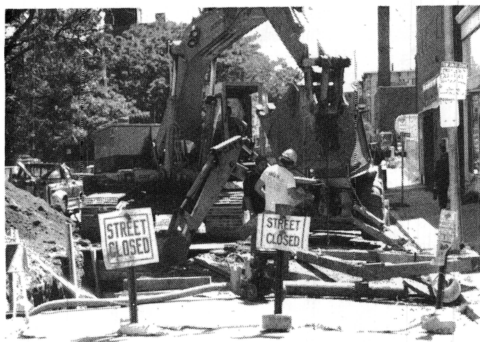
Sewer replacement — Prospect Street at Bishop Allen Drive.
