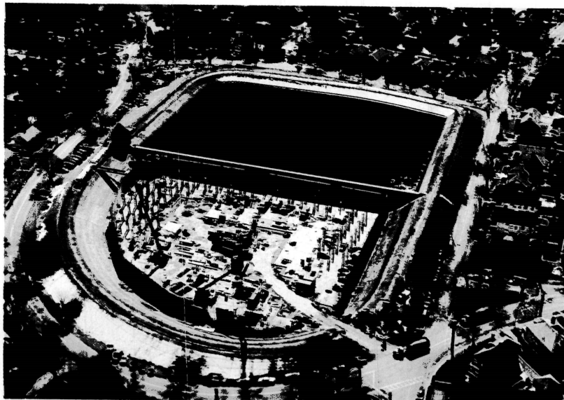
March, 1990 — Construction of the North Tank being performed while the original South Basin was still providing uncovered treated water to the city.
