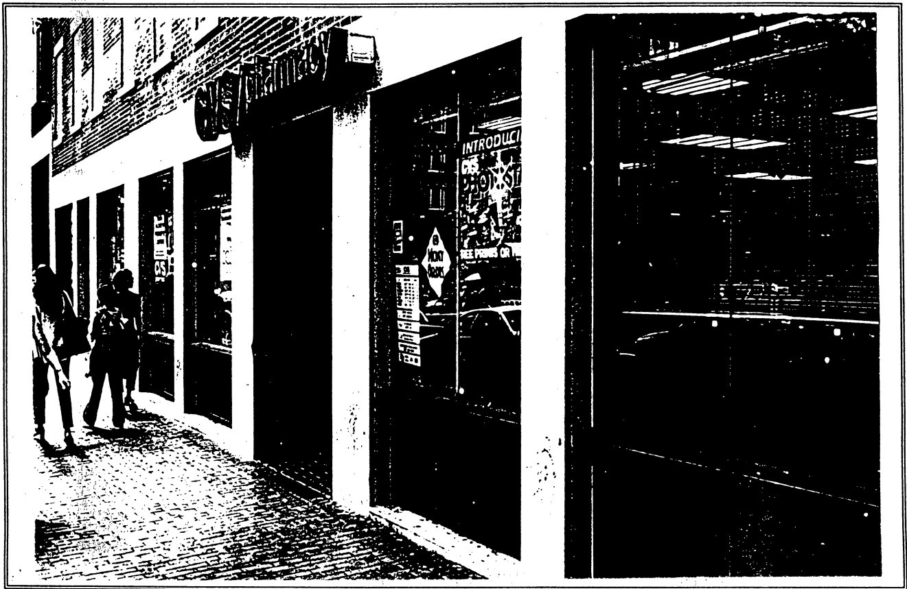
Figure 5. College House storefront, 1999.
