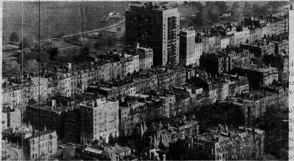
Back Bay, Boston. Rehabilitation of existing housing stock is stressed by densely settled communities.
