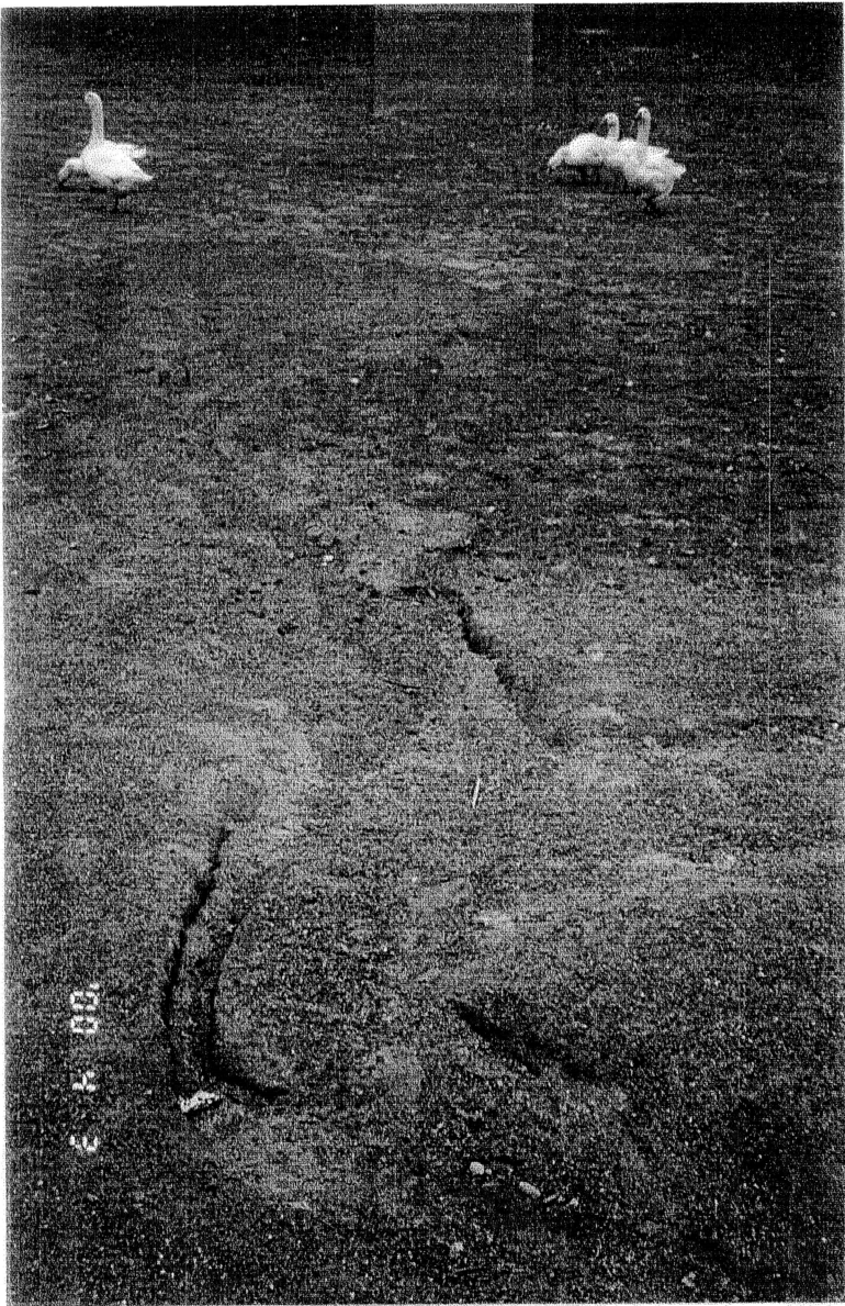
Erosion from walkway
