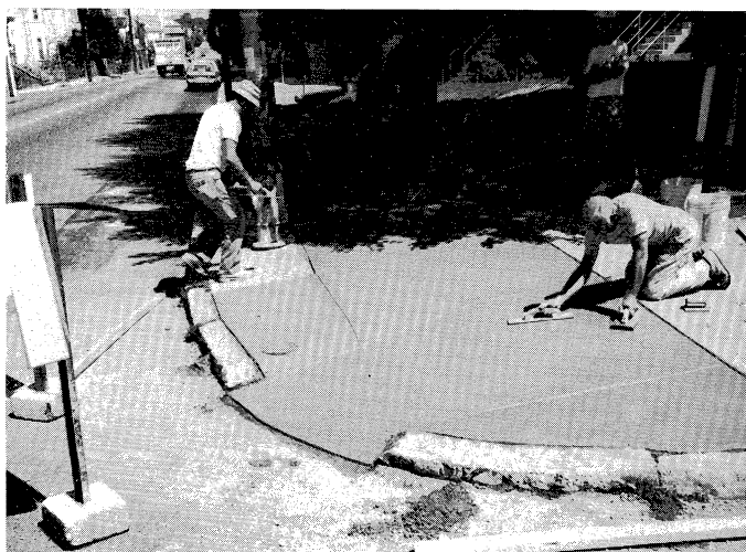
Preliminary "floating" of new concrete pedestrian ramp and sidewalk.
