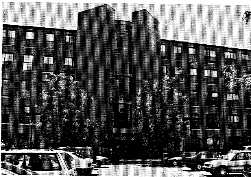
The former Henderson Carriage Factory was rehabilitated for use by a variety of occupants, including a restaurant, a bank, and several small firms.
