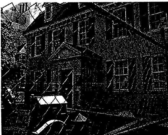
Construction Progress at CCAE
