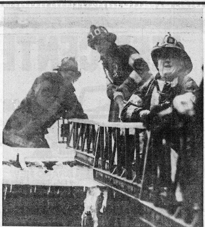
Boston firemen erect and man ladders (top) to fight a $50,000 fire that swept the former Astor Theater on Tremont Street, opposite the Boston Common. Firemen were hampered by parked cars (bottom), blocked hydrants and the old marquee attached to the front of the four-story building. One fireman suffered a leg injury in the firefighting operation.
