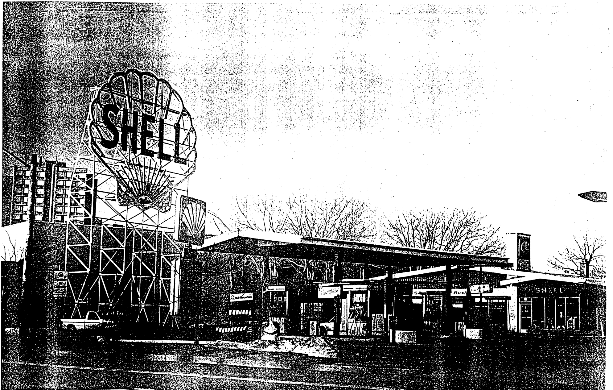
Shell Sign 187 Magazine Street Southeast Elevation April 1990
