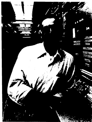
Central Office Repairman George Montville is at the control panel of the Worcester, Massachusetts, Electronic Switching System (ESS). Placed in service in October 1976, the Worcester ESS serves 63,000 customers. This equipment is capable of handling 230,000 calls an hour. ESS also allows us to offer custom calling features such as call forwarding, speed calling and three-way calling.
