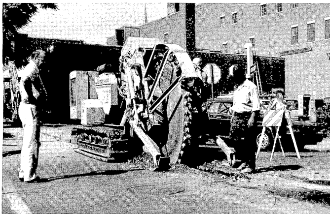
Inspection of underground Cable/TV Installation throughout the City.
