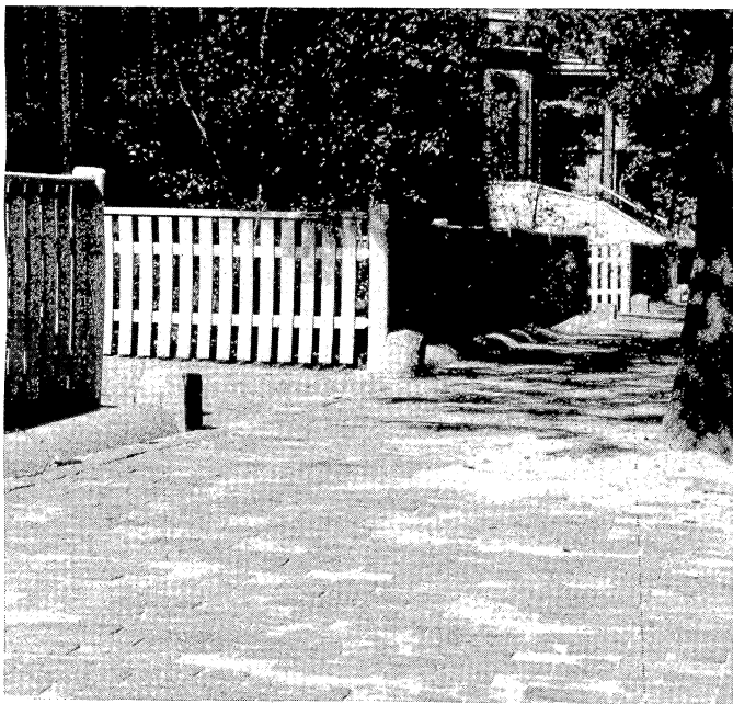
New brick sidewalk along Harvard Street.
