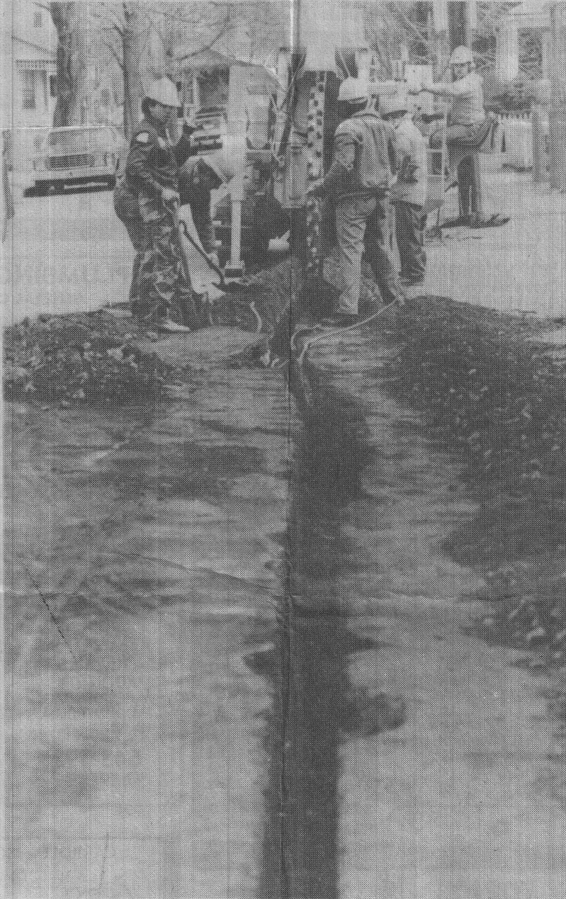
LAYING THE LINE—American Cablesystems workers were busy laying cable on Blake street last week. (Staff photo by Carolyn Hine)
