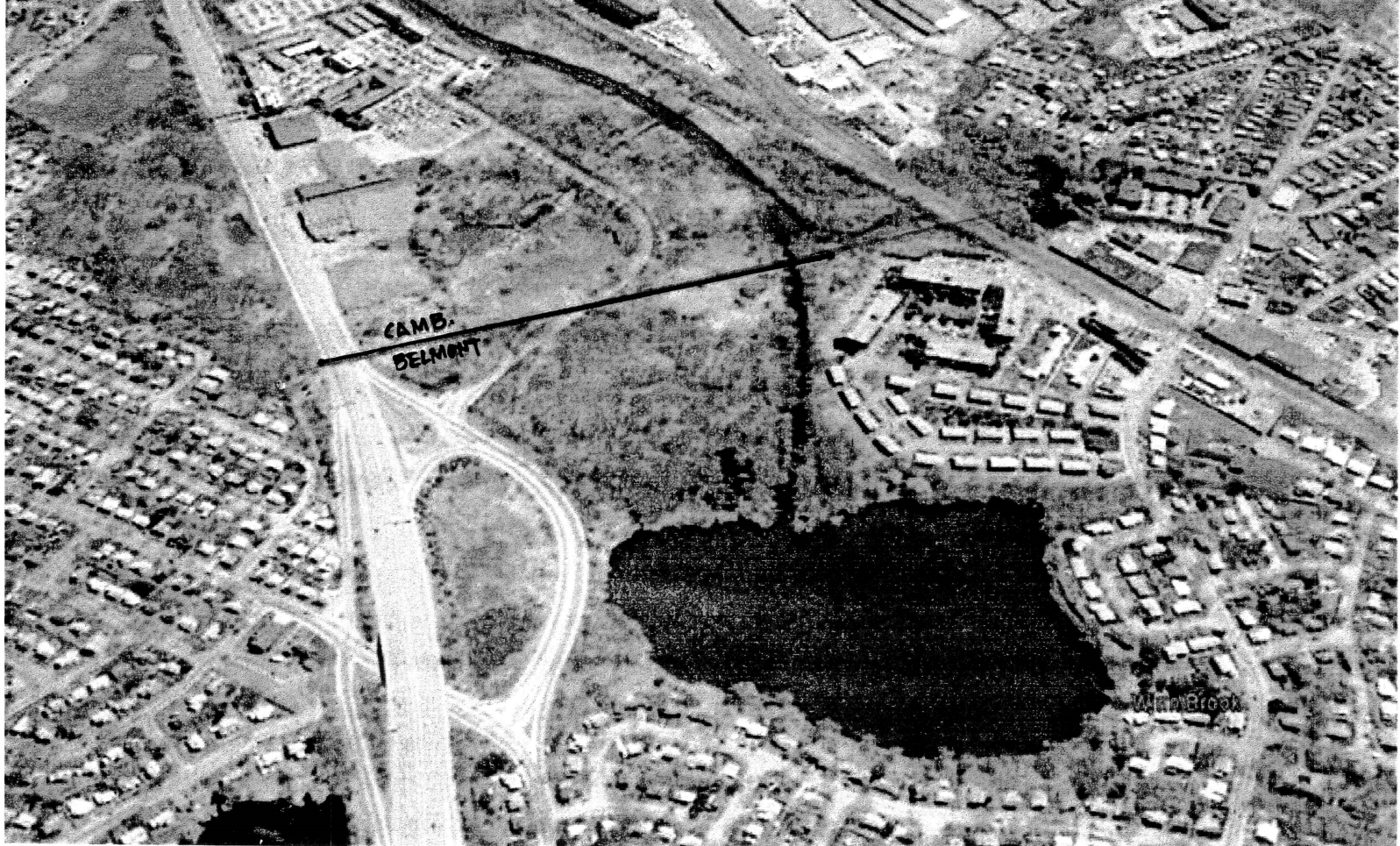
Computer aerial view looking east - existing silver maple forest in center of photo
