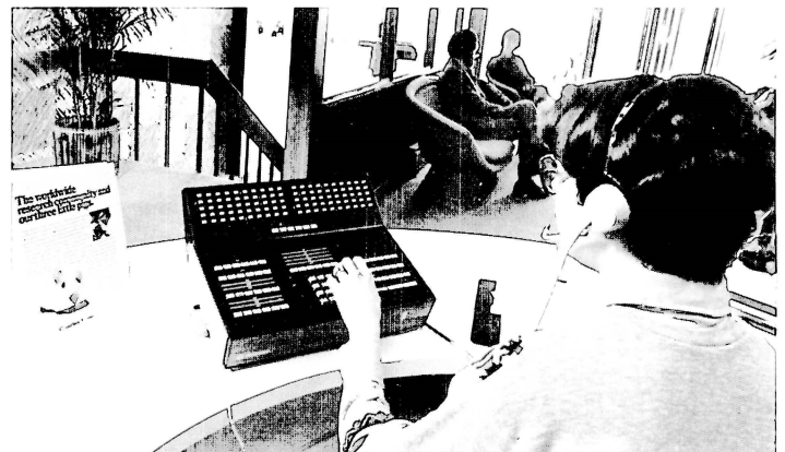
A laboratory facility in Wilmington, Massachusetts, chose the Dimension® 2000 PBX as the answer to its communication needs because it provided them with the flexibility needed to change and grow. The solid-state equipment can be programmed like a computer to perform specialized business functions.
