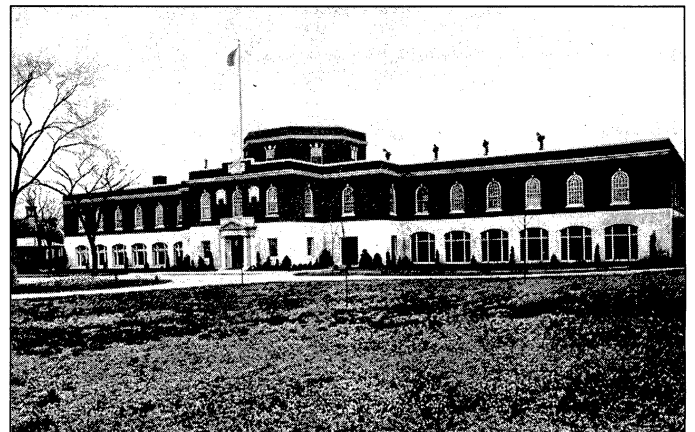
Water Treatment Plant as constructed in 1924
