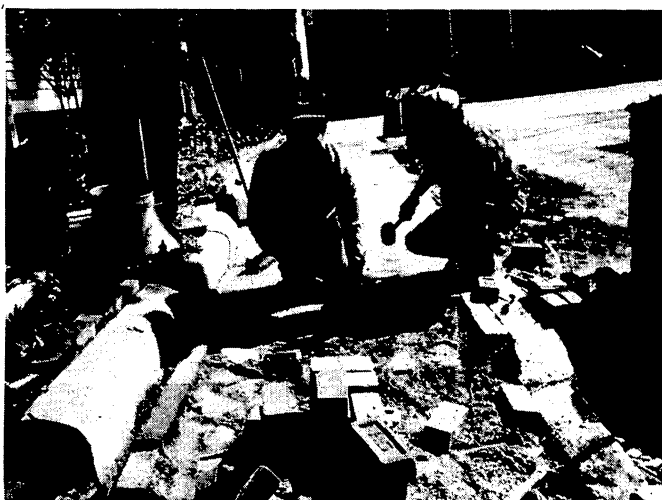
Laying down a new brick sidewalk on R.C. Kelly Road.
