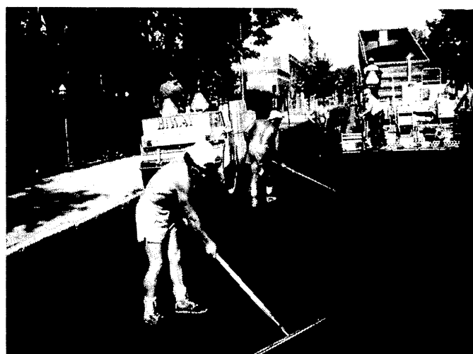
Grinding and overlaying a new surface on Broadway.
