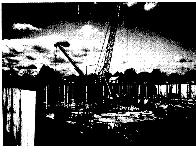
South Basin Tank under construction.
