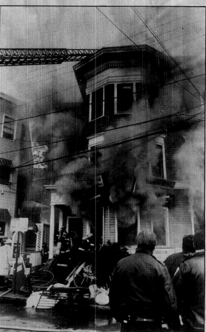
FOUR-ALARM BLAZE — Cambridge firefighters responded to a four-alarm fire at Elliott and Winthrop streets at 7:09 Wednesday morning. The fire damaged two buildings, 16-18 Elliott St. and 98 Winthrop St. The Elliott street building, a four-story commercial and residential structure which houses the Ta Chien and Roka restaurants, sustained the greater damage. Residents were evacuated. The Winthrop street building includes the Henry IV restaurant. The fire department is conducting an investigation into the source of the blaze. (Staff photo by Cheryl Miller)
