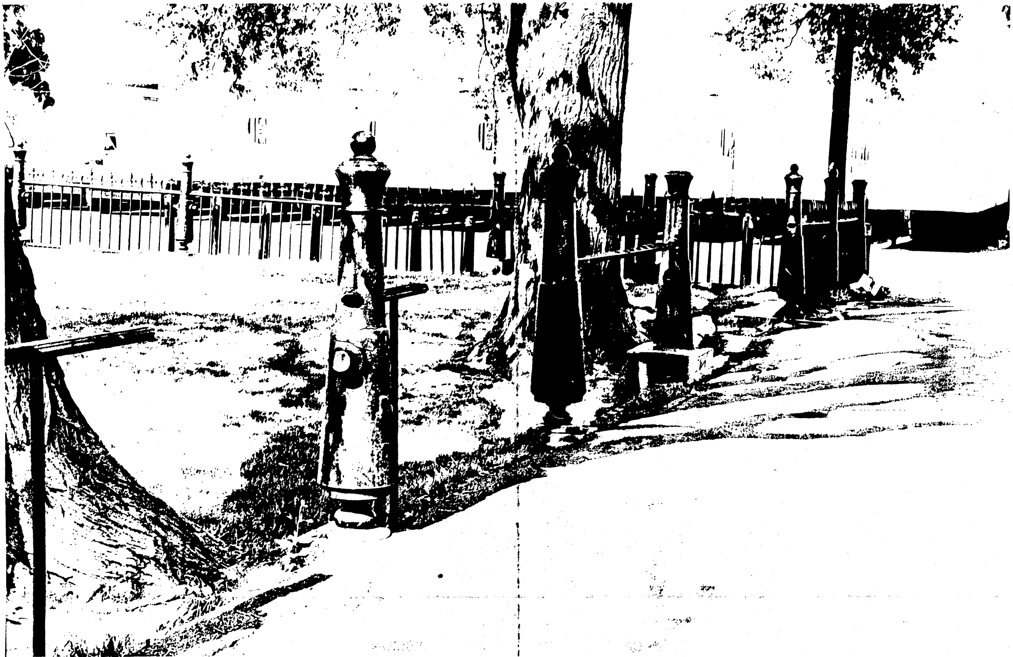
Fort Washington in 1975, showing deterioration of fence.
